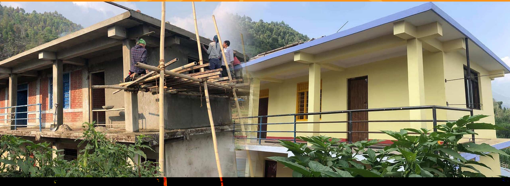
The Sarsyu School during construction and after completion.
